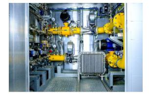
The spectrometer for the infrared active components of natural gas and the thermal conductivity sensor for measuring hydrogen are installed in a natural gas bypass system belonging to Fraunhofer ISE. The measuring device is housed in an explosion-protected case with fins for faster cooling (photo, bottom right). © Holger Kock/Fraunhofer IPM
