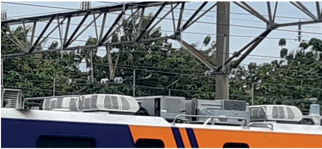
The CIS installed on a train: The system is located between the two white air conditioning modules.
